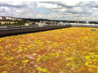
efficient stormwater management with low maintenance needs. Extensive greenroofs are very cost efficient.
