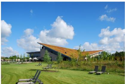
content varies from the ridge to the eave (lowest edge of the roof). It is the task of the designer to make adjustments in the green roof system accordingly (e.g. drainage, thickness of growing media plant varieties etc.). Recent failures of sloped green roofs in the United States showed that many of designers are not aware of this unique situation. This is most unfortunate and the amazing design that they had in mind rarely develops into a successful and lasting one.
