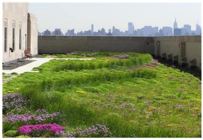
to host a richer ecology. Though higher in maintenance, this green roof system also provides the potential for a formal garden effect.
