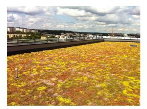
An extensive green roof system is characterized of its vegetation, ranging from sedums to small grasses, herbs and flowering herbaceous plants, which need little maintenance and no permanent irrigation system. The growing medium depth for an extensive green roof system is typically 6 inches or less. These systems are ideal for efficient stormwater management with low maintenance needs. Extensive greenroofs are very cost efficient.
