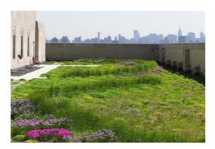
A semi-intensive green roof system is characterized by small herbaceous plants, ground covers, grasses and small shrubs, requiring moderate maintenance and occasional irrigation. A typical growing medium depth for a semi-intensive green roof is 6 to 12 inches. This system is able to retain more stormwater than an extensive system and provides the potential to host a richer ecology. Though higher in maintenance, this green roof system also provides the potential for a formal garden effect.
